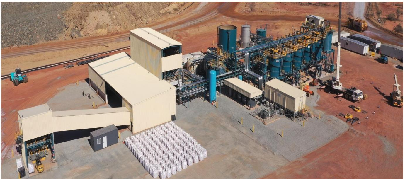
**Figure 1. Stage 1 sulphide flotation plant.**
