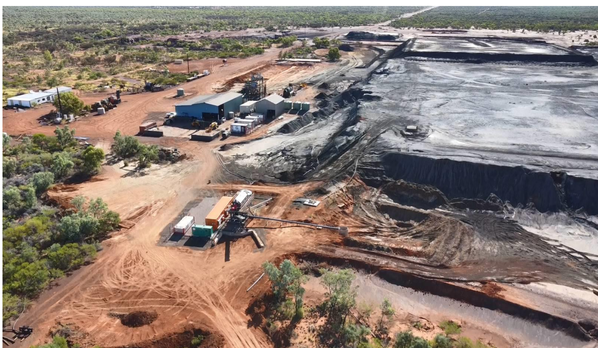
Peko Magnetite Plant, next to Peko circa 3.75MT stockpile, with Screw-press (for drying tailings) in centre foreground.
