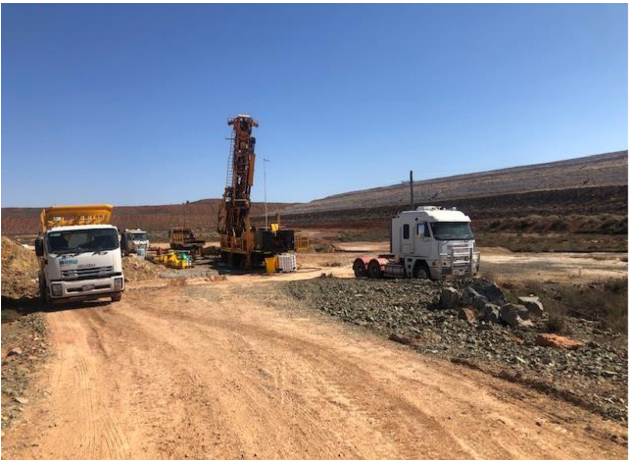
Figure 8: Drill Rig at Wiluna Site
