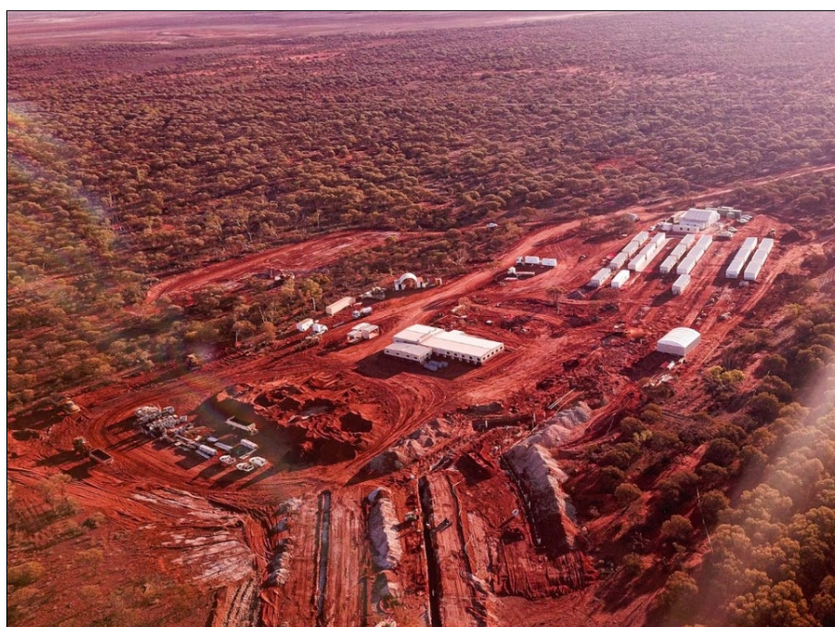
Figure 2: Bellevue camp construction showing the progress to date with 80 of the 330-person camp landed and installed with the dry mess installation in the foreground.
