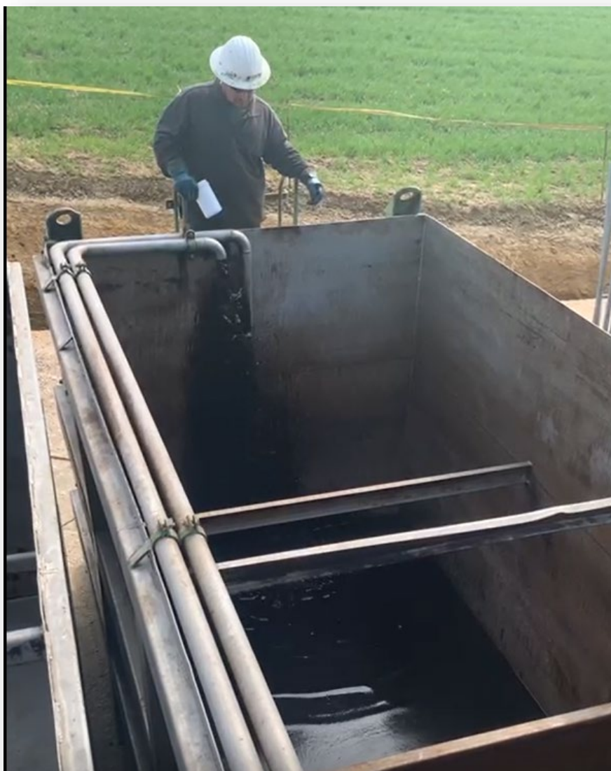
Photograph of Anshof-3 Production Test
