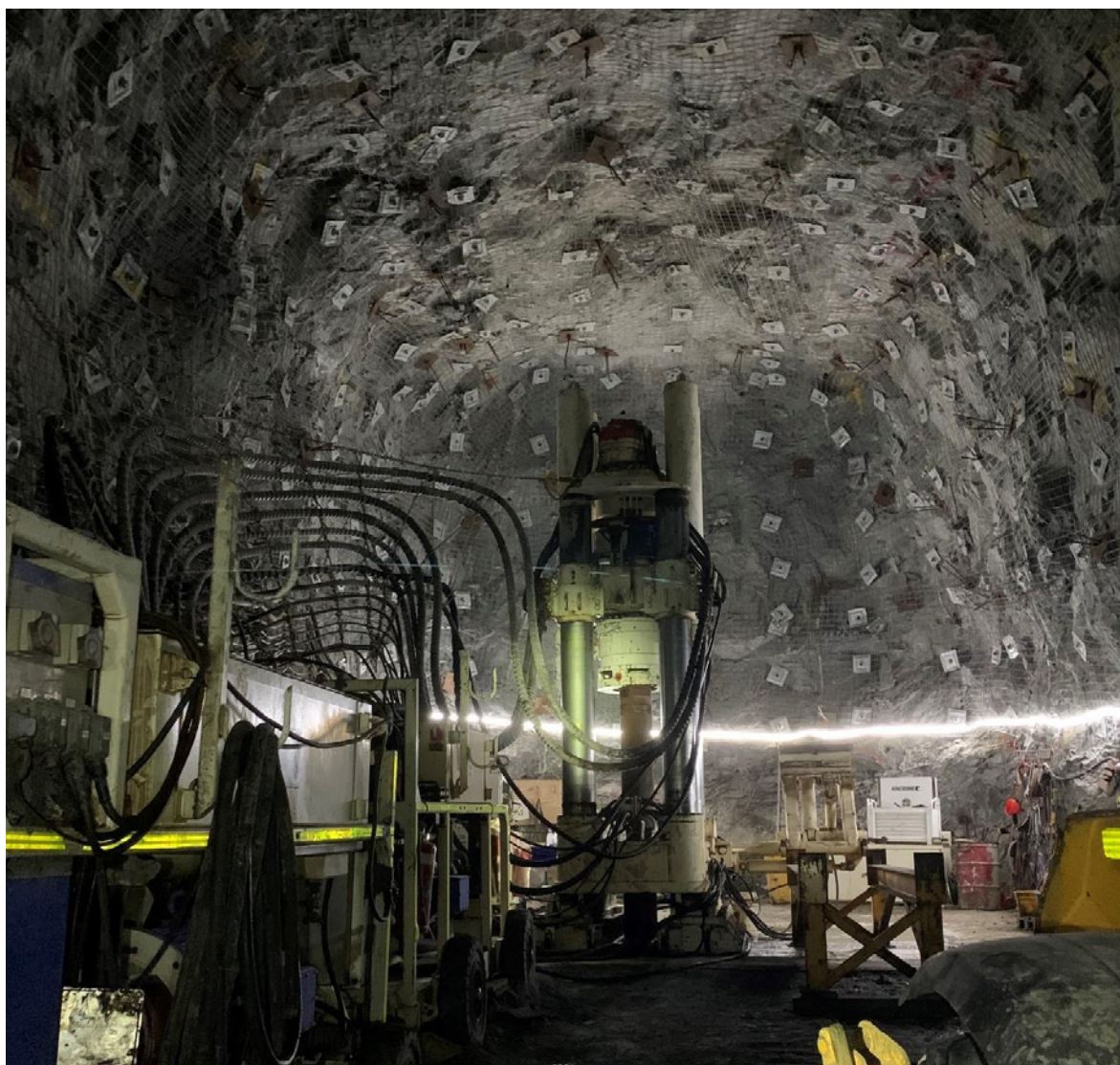
Figure 4.9: Raise boring of the second leg of the hoisting shaft
