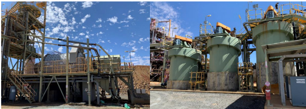
Figure 4.4: Cosmos nickel concentrator - existing mill and roughers
