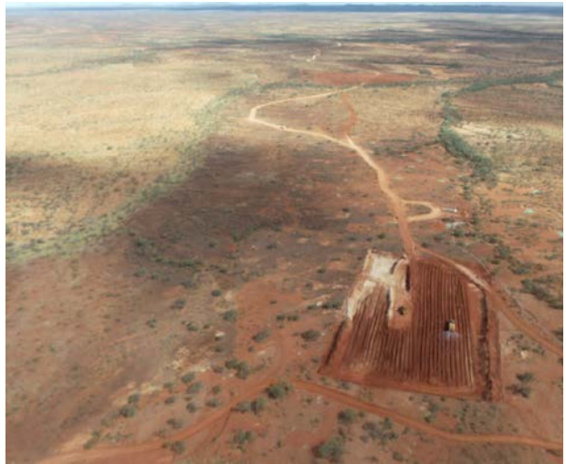
Borrow Pit material for access roads
