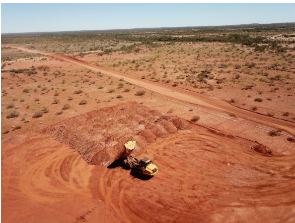
Placing of fill material at the 300-bed village site
