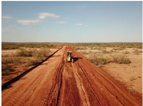
Haul Road construction
