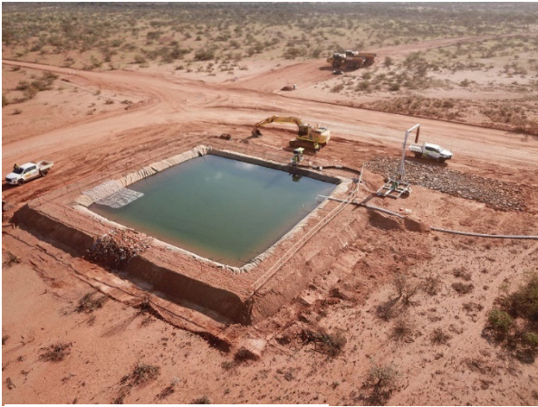
Turkey's Nest Construction
