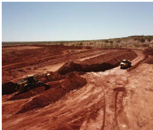
Extraction of borrow pit material
