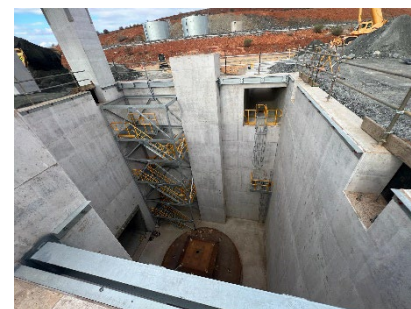
Shaft sub-brace concrete and steel-work
