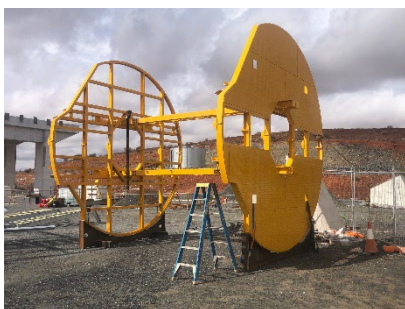
Shaft sinking stage
