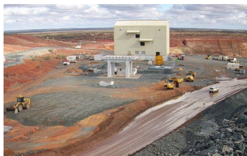
Shaft terrace layout with box-cut backfilled
