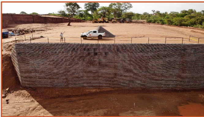
Figure 4: ROM Retaining wall (left) and thickener foundations (right).
