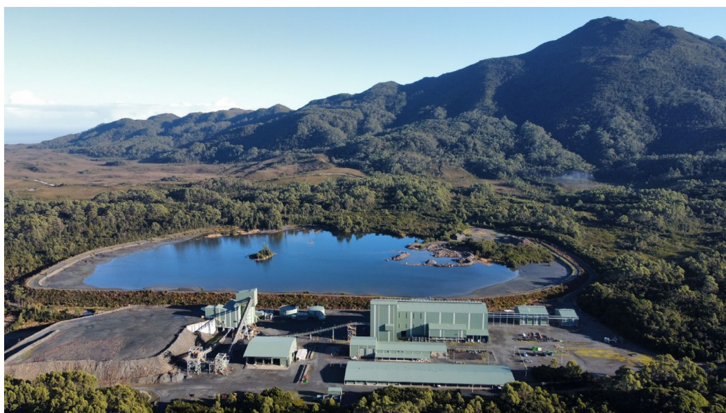
Figure 3. Avebury processing plant and site infrastructure
