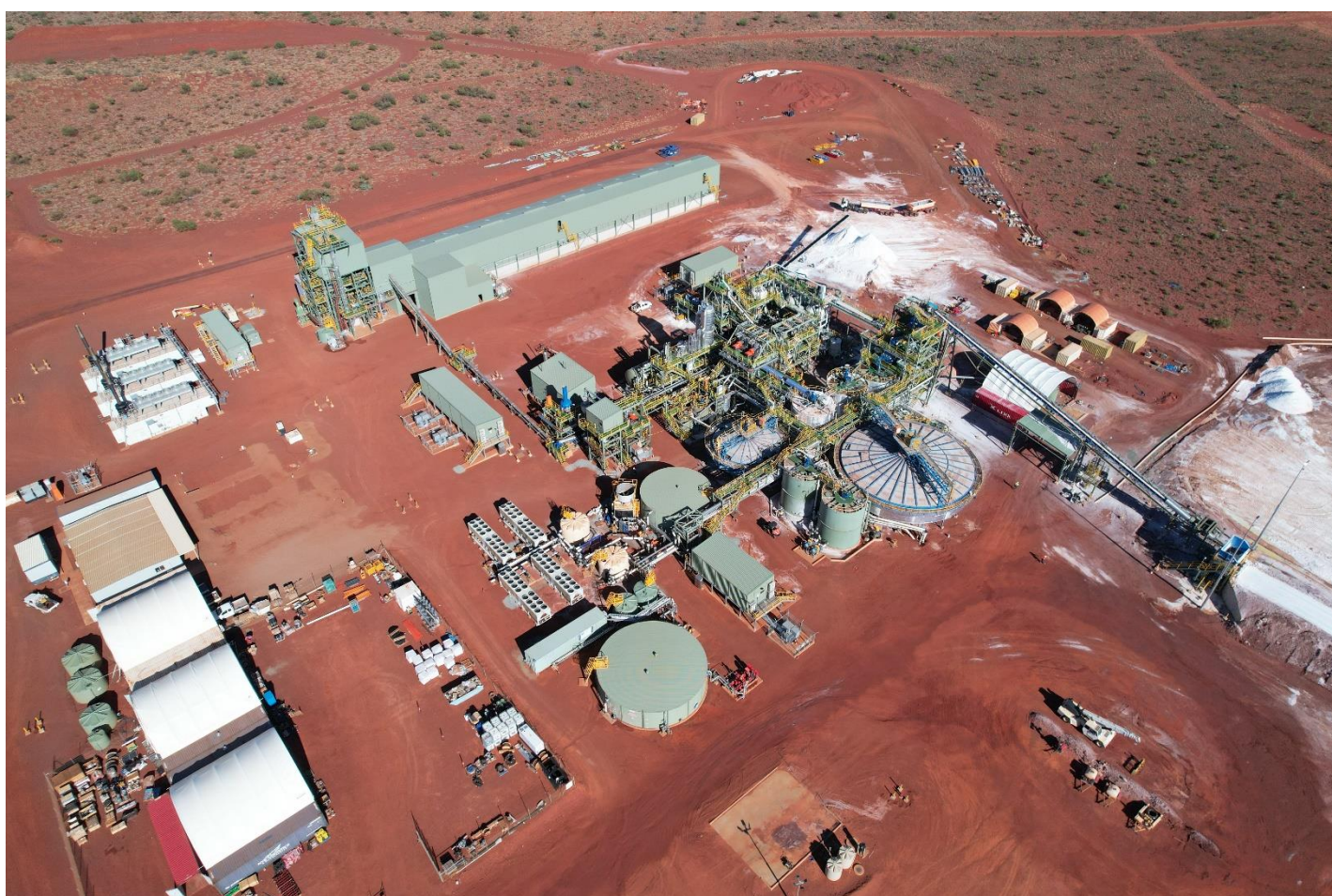
Beyondie Sulphate of Potash Purification and Compaction Plants
