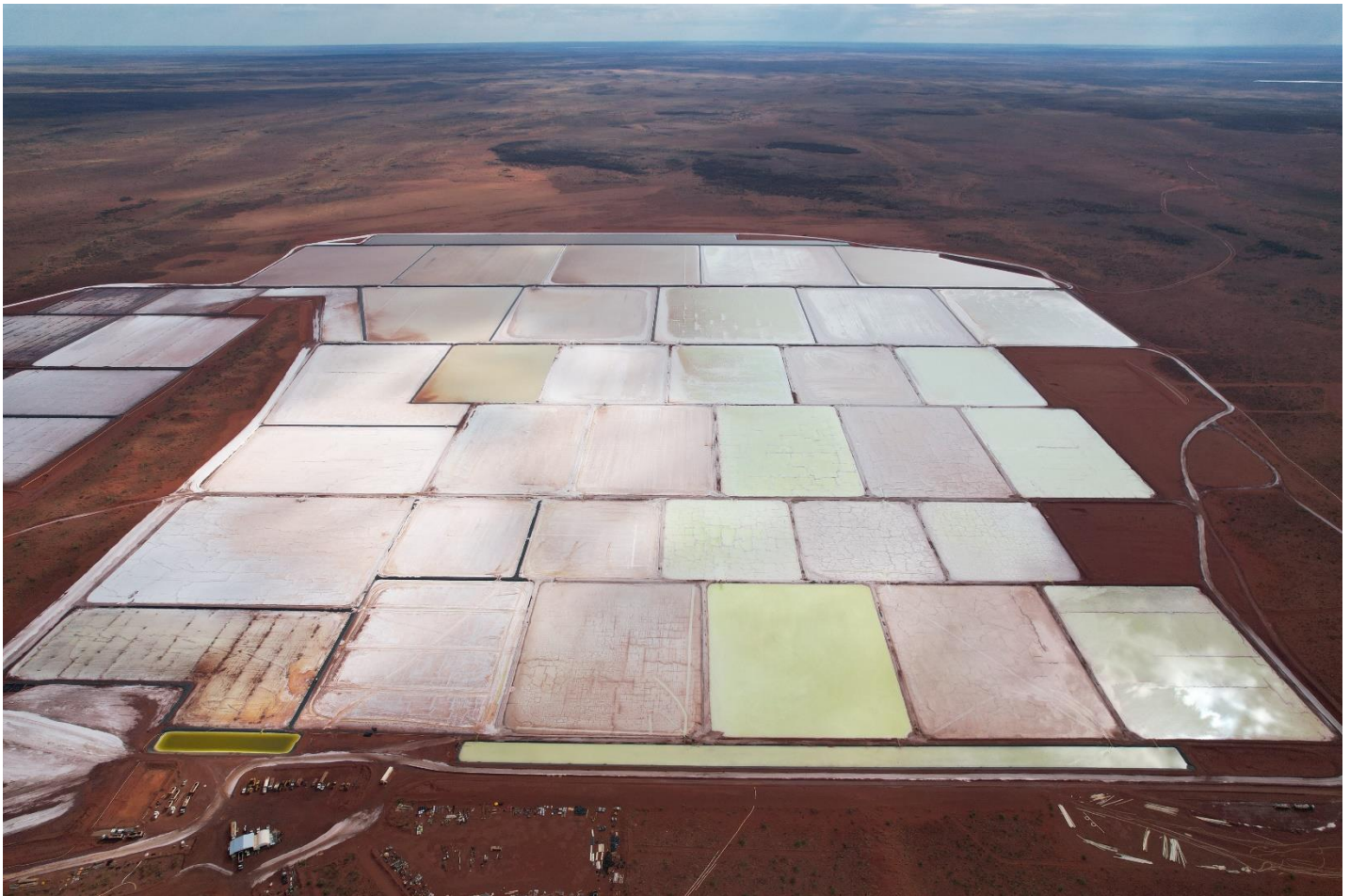
Aerial image of Beyondie primary evaporation pond trains (as at 28 March 2022)
