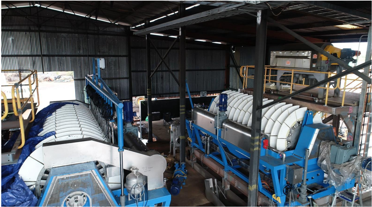
Commissioning of final stage of plant (dewatering ceramic disc filters) near completed
