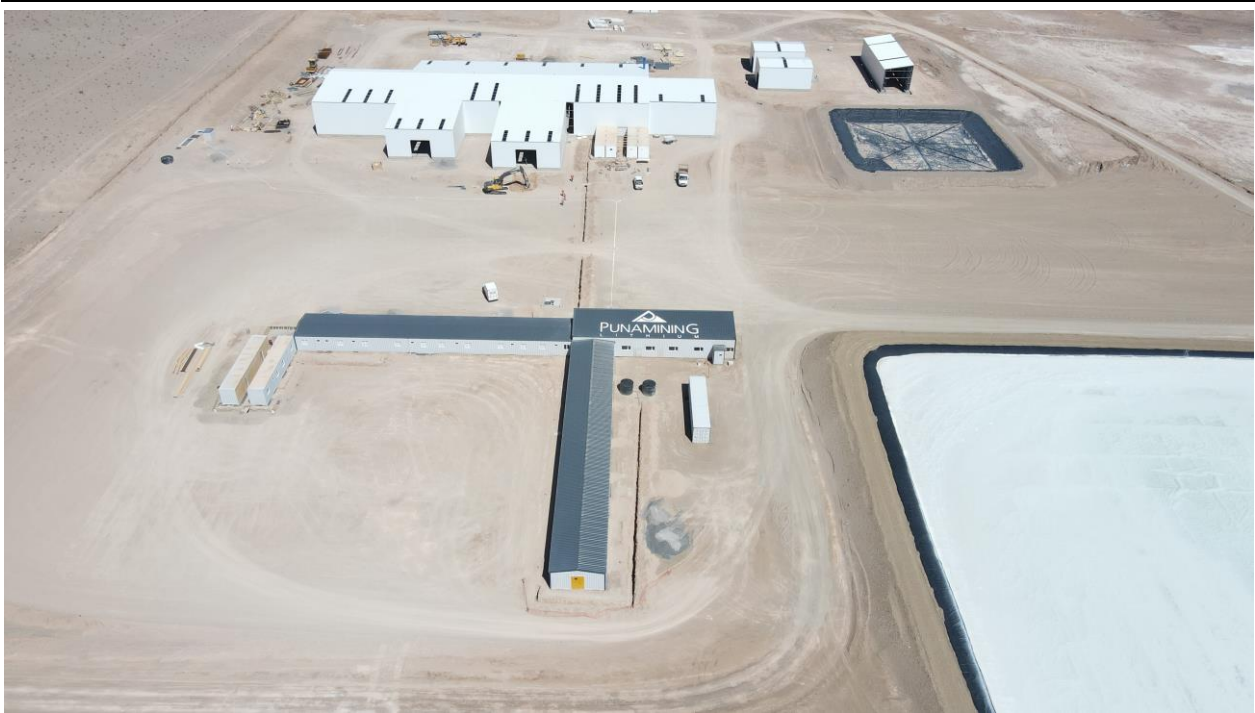
Figure 5. Rincon Lithium Project – 2,000tpa Operation Site Works
