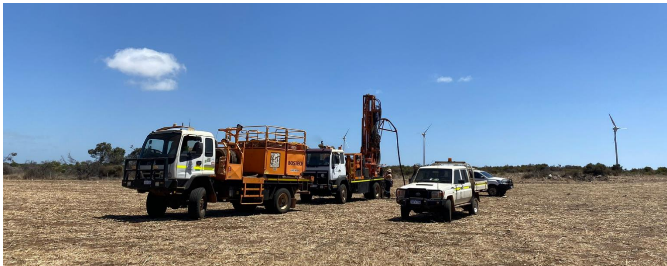
Figure 4: Bostech drilling rig on site
