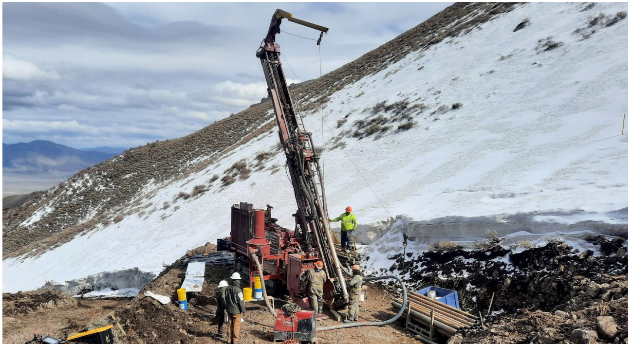
Figure 3. RC percussion drill rig on site drilling the first hole at Star Canyon, Nevada.
