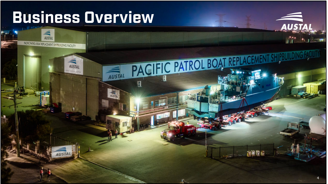
A Guardian Class Patrol Boat being transported from Hope Valley Road to waterfront for Launch.
