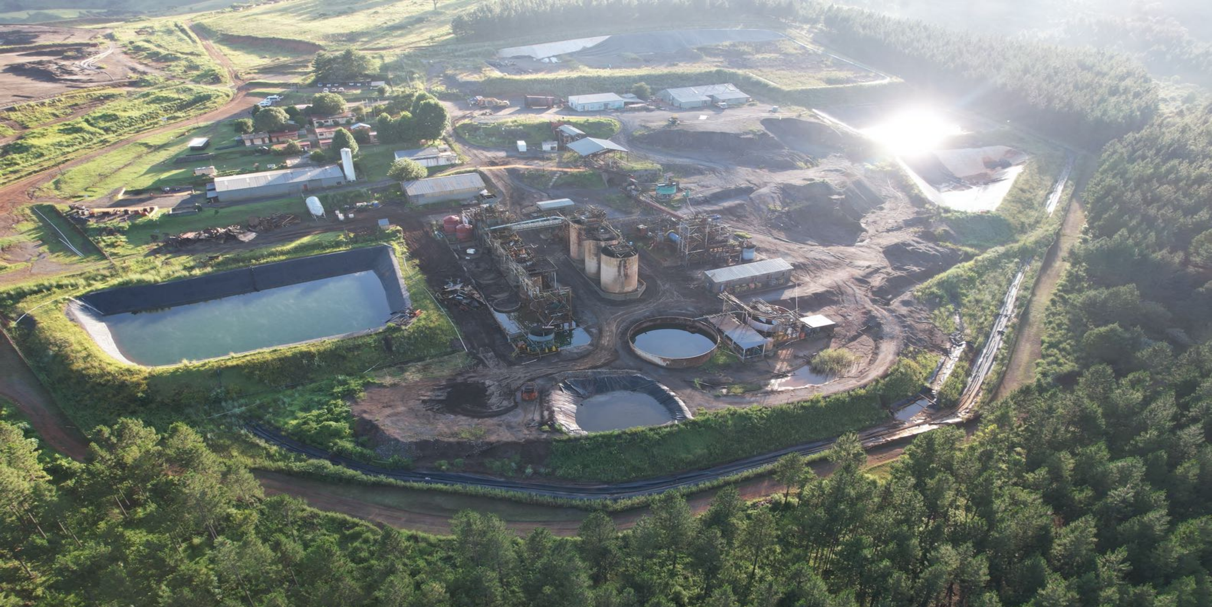
OLD PLANT DEMOLISHED READY FOR NEW PLANT BUILD (APRIL 2022)
