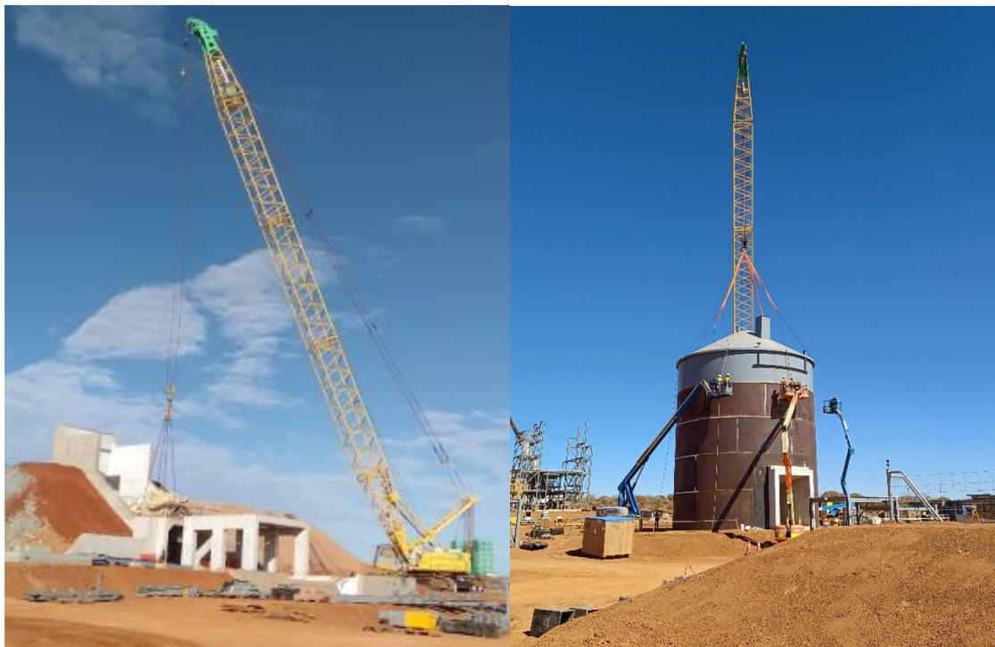
**Figure 1** – Lifting of the primary jaw crusher and fine ore bin top into position.
