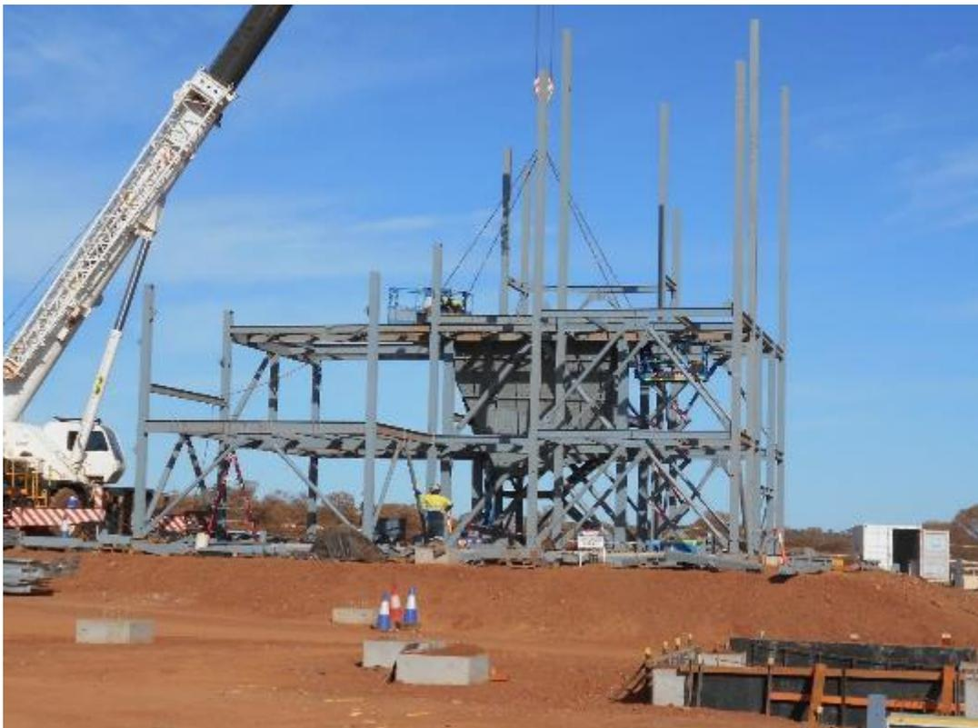
**Figure 7** – Crushing screening area steelwork.
