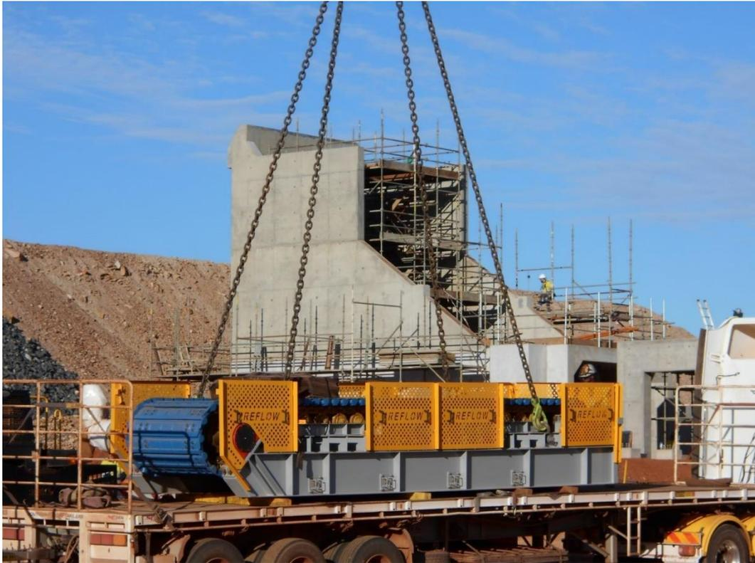
**Figure 6** – Arrival of primary crusher feeder.
