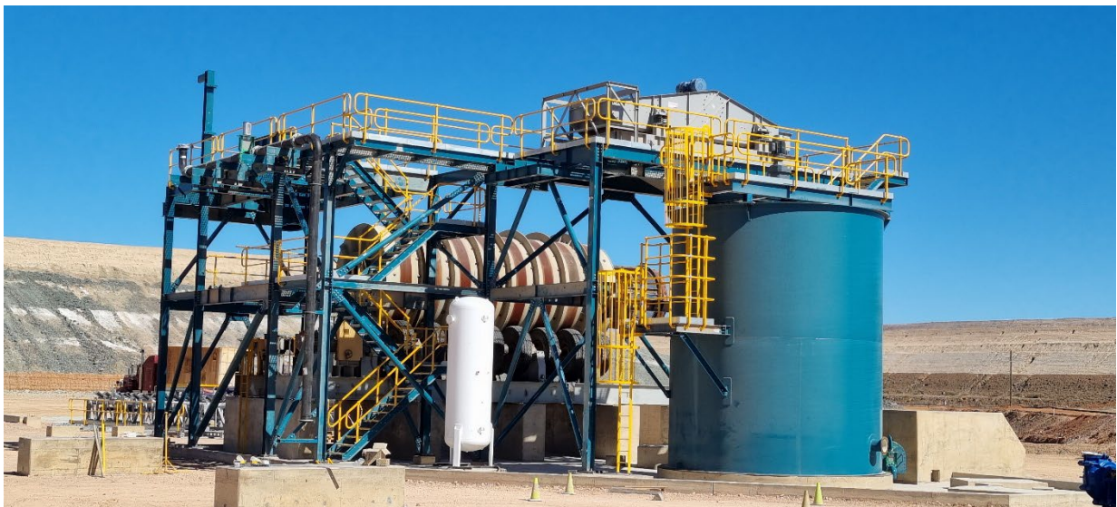
Figure 2: WilTails Plant Construction Progress
