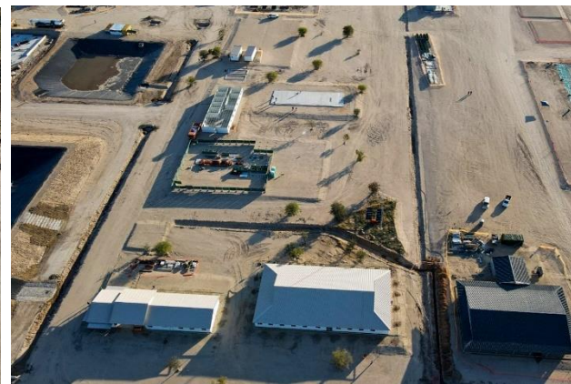
Process Plant and Mining Offices Overview
