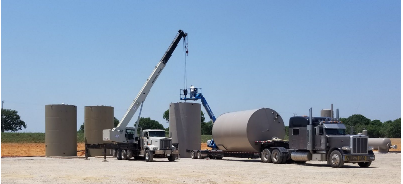
Figure 1. Production facilities arriving on location and being plumbed in
