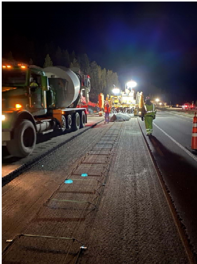
Figure 2- Placing portion of the concrete pavement at night
