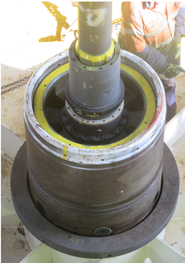
Downhole drilling assembly and installation within the well head housing on the mudmat
