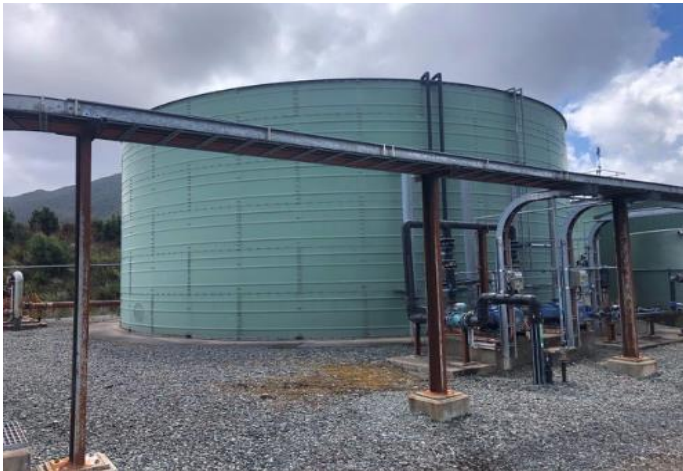
Water Section Asset 1H - 7 - Water Tank
