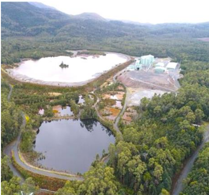
Figure 4 Avebury Mine site
