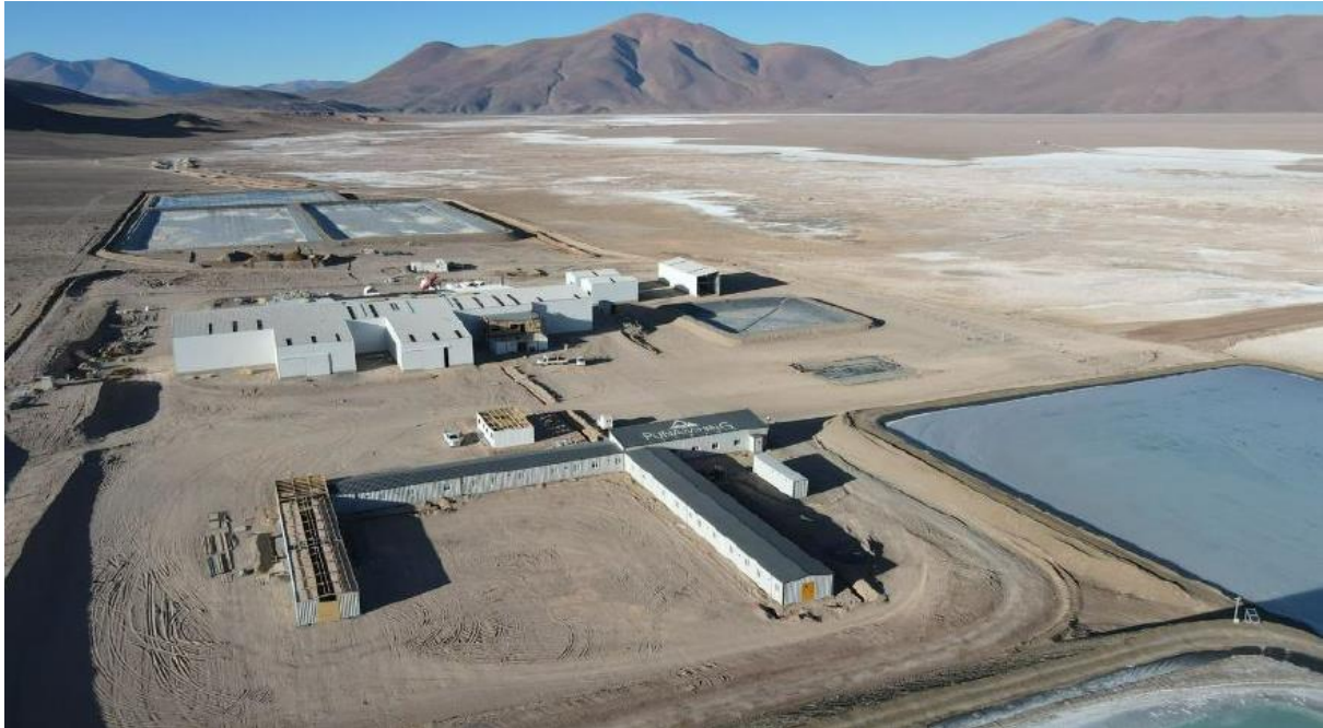
Figure 2. Rincon Lithium Project – 2,000tpa Operation Site Works
