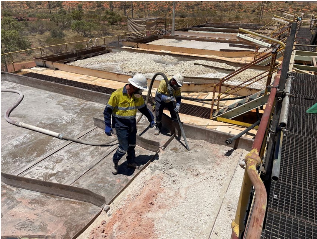
Image 2 / SX Mixer Settler clean-up top level
