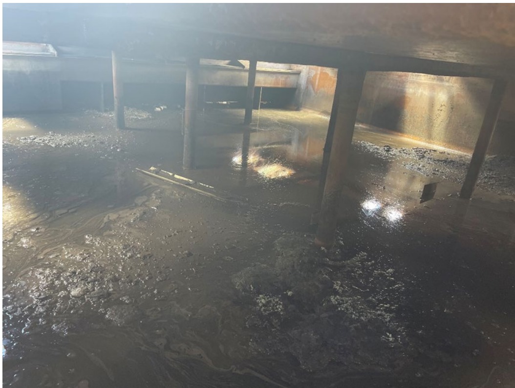
Image 3 / SX Mixer Settler cleanout lower level – before
