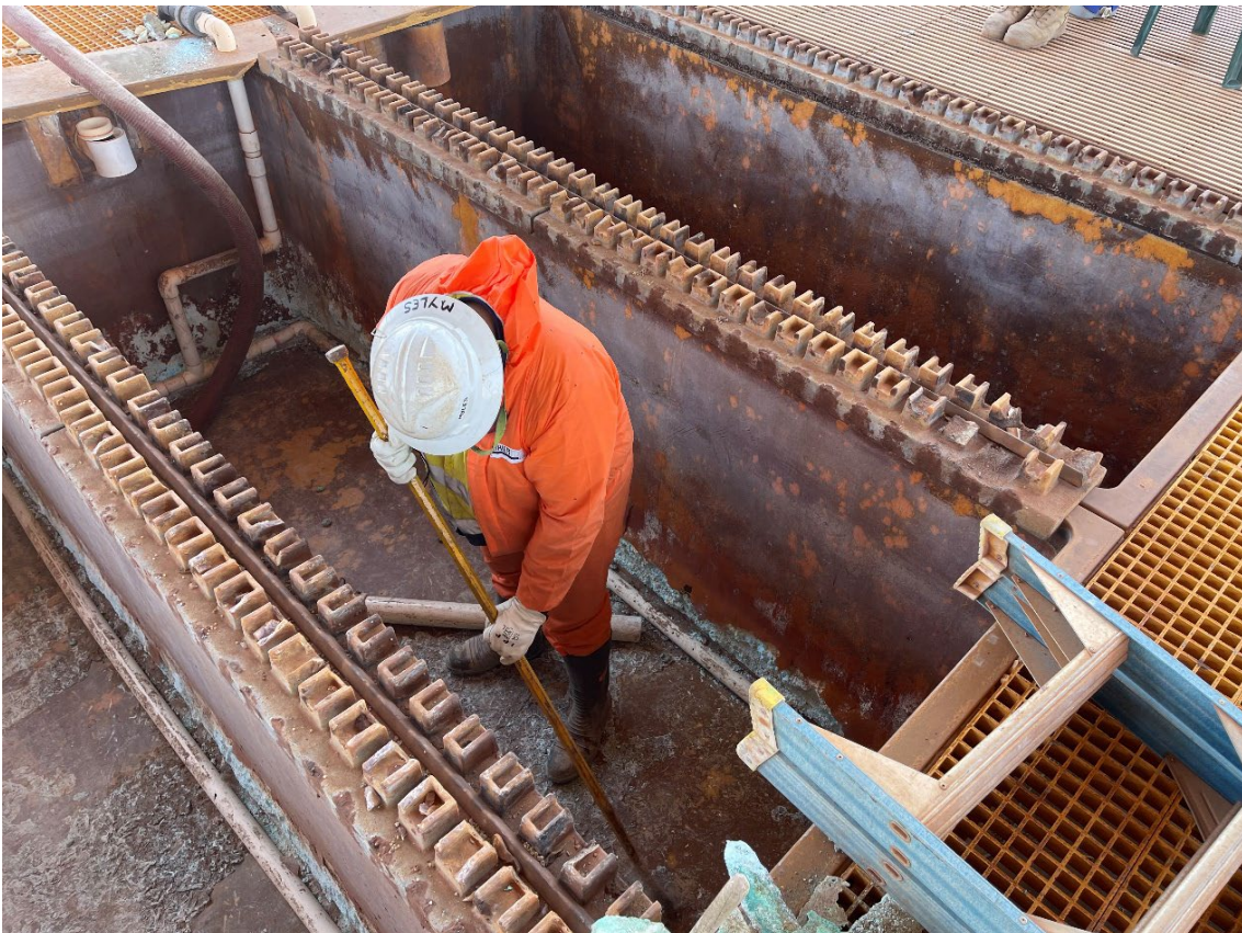
Image 7 / Cleaning out EW Cells post Hydro testing
