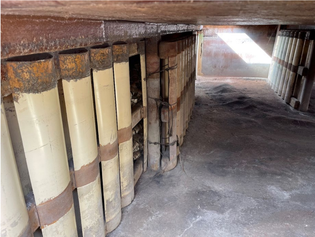
Image 4 / SX Mixer Settler cleanout lower level – after
