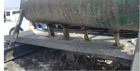
Large amount of salt coming out of the Paradox Lithium Project Long Canyon Long Canyon #2 well (an indicator of the presence of brine) on approaching the start of Mississippian Zone, at a depth of 2346m.
