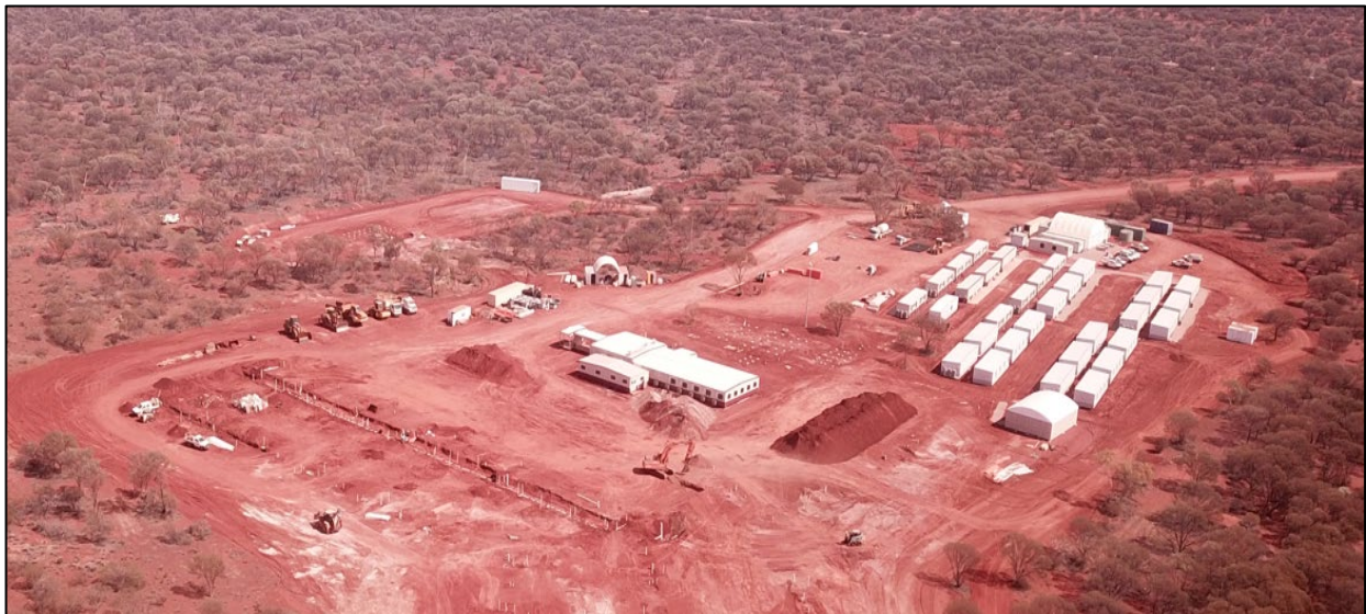
Figure 9: Village Construction Progress (as of 21 April 2022)
