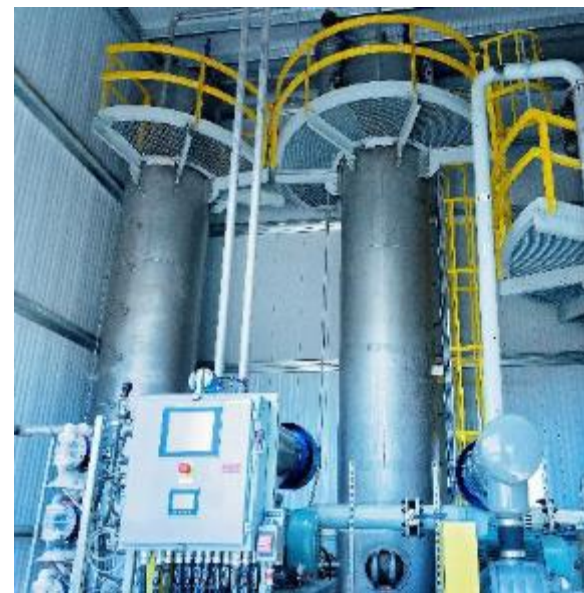
Operational H2Sweet Sulfcats treating unit installed at Calima’s 2-29 Brooks battery
