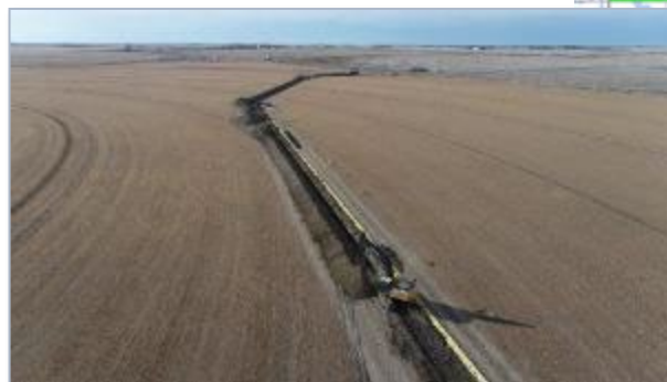
Construction of the Bantry north-south dual-pipe interconnect which is expected to positively impact CO 2 e emissions.
