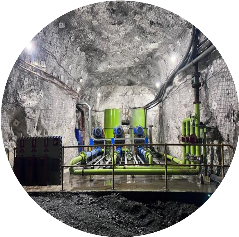
Underground Water Pumping Station
