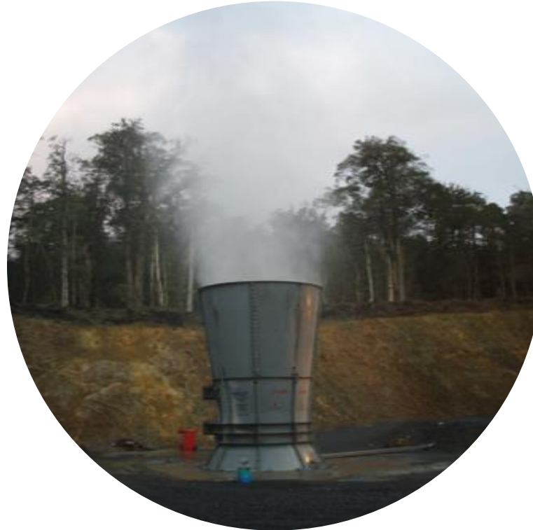
Avebury No.2 Vent Rise
