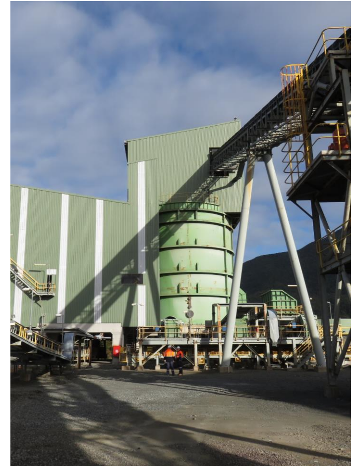
Crusher House and Fine Ore Bin
