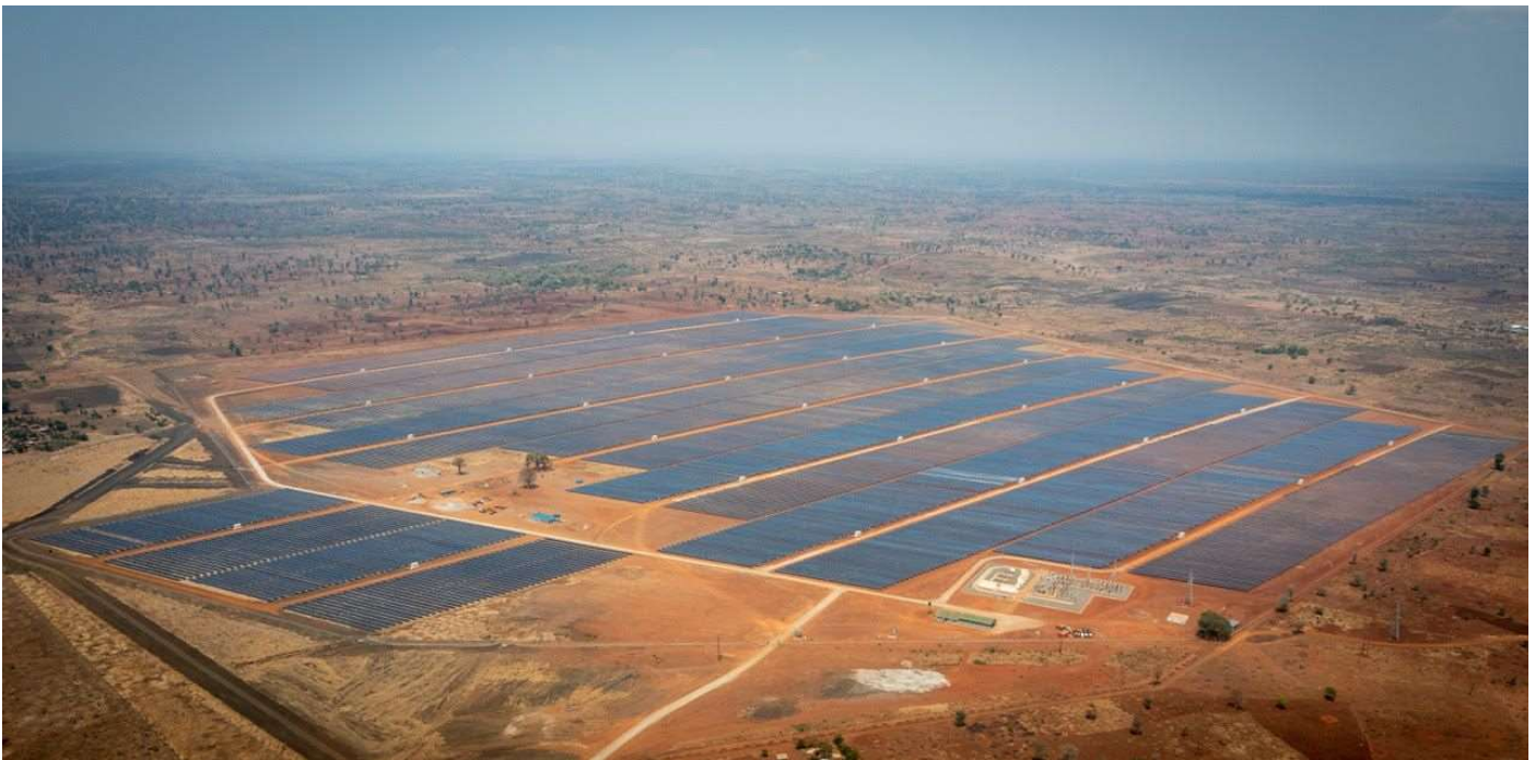
Figure 28: 60MW Salima Solar Power Plant in Malawi recently constructed and commissioned by JCM (source: JCM)
