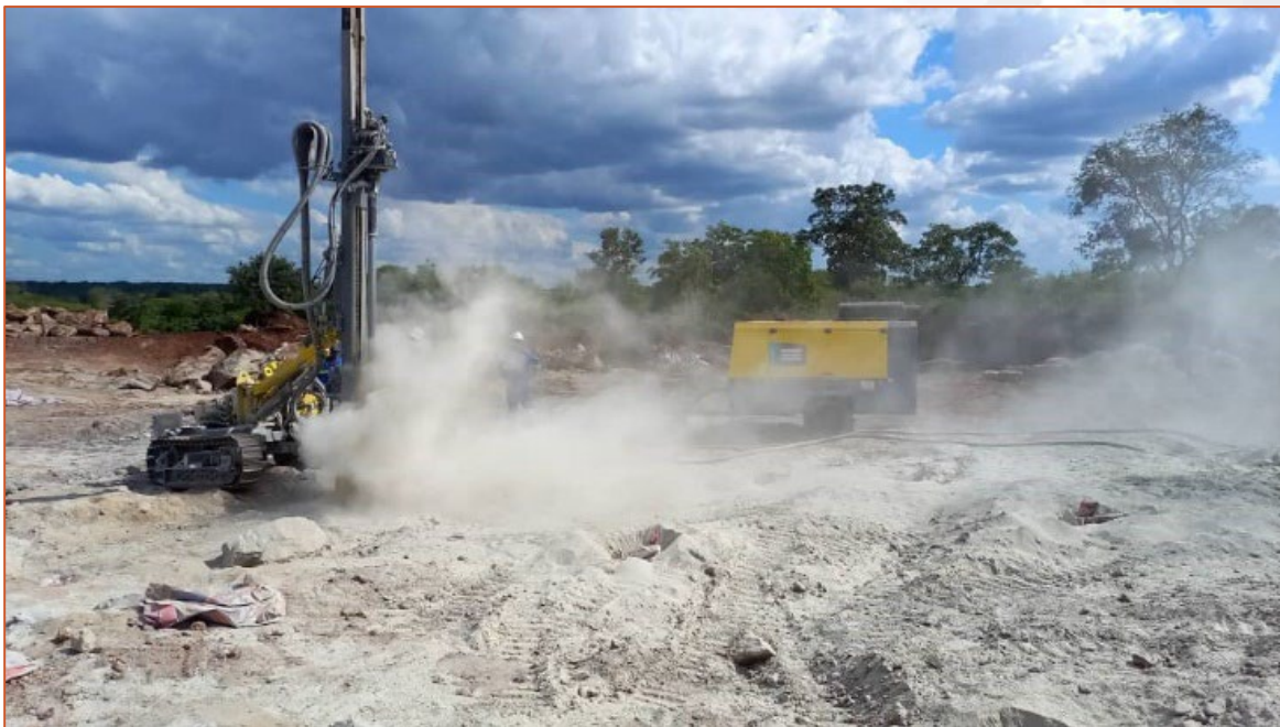
Figure 7: Drilling in preparation of the first blast.
