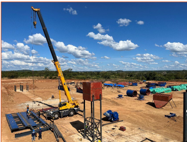
Figure 5: Steelwork construction on site using the Lindi Jumbo 55-ton crane (left) and transport of an assembled section of the fine-ore bin for installation (right).
