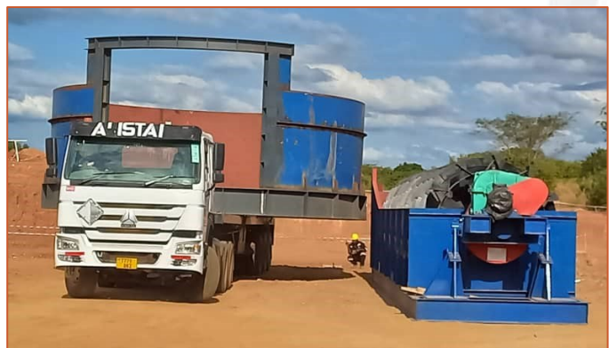
Figure 5: Steelwork construction on site using the Lindi Jumbo 55-ton crane (left) and transport of an assembled section of the fine-ore bin for installation (right).
