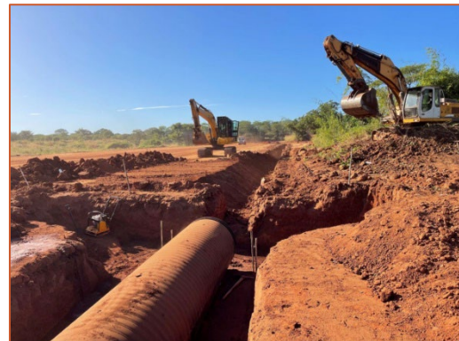
Figure 1: Oblique view from the south of the TSF. Clay filled cut-off keys around the TSF footprint are clearly visible (left). Excavation of the stormwater cut off trench at the TSF (right).
