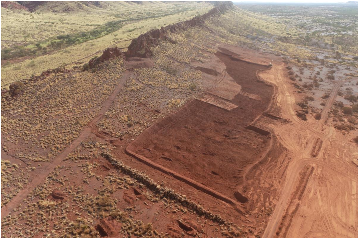
Figure 1: Excavation of Detritals Iron Ore on Northern Slope of Paulsens East Hematite Ridge
