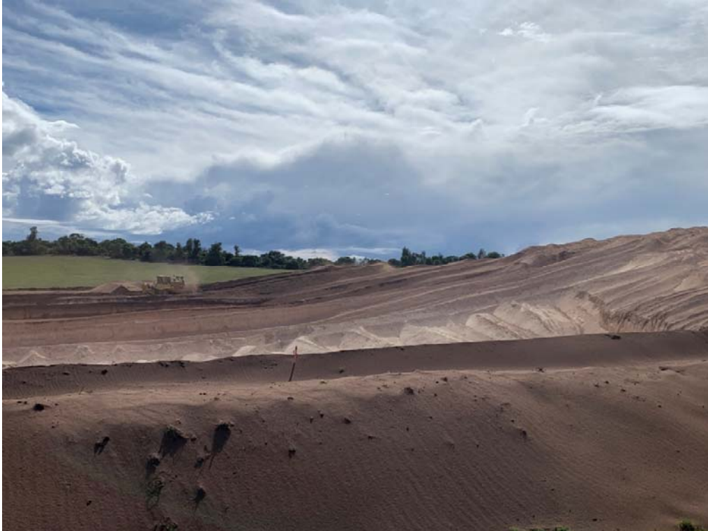
Figure 2 Topsoil Removal and stockpiling for future rehabilitation
