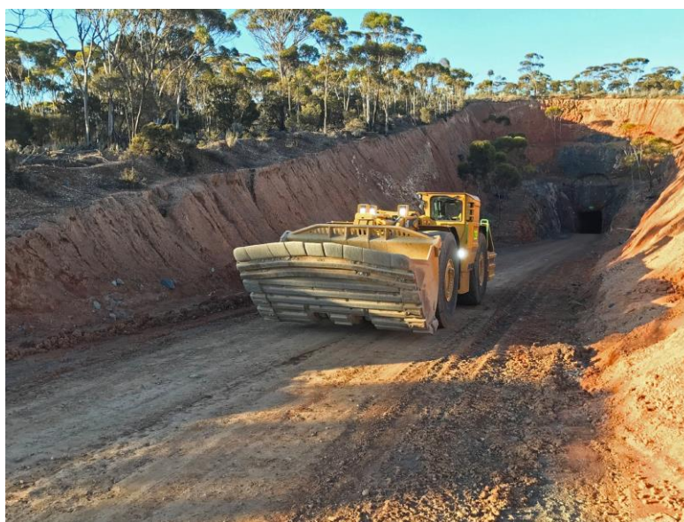
Image 4: Bogger exiting the OK Underground Mine Portal
