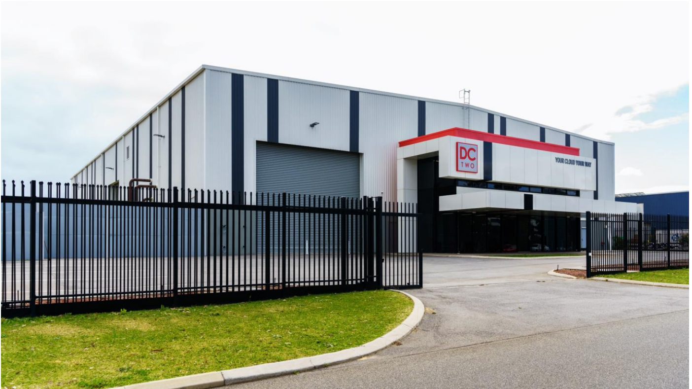
DC Two's Tier III Design Accredited data centre – Bibra Lake
