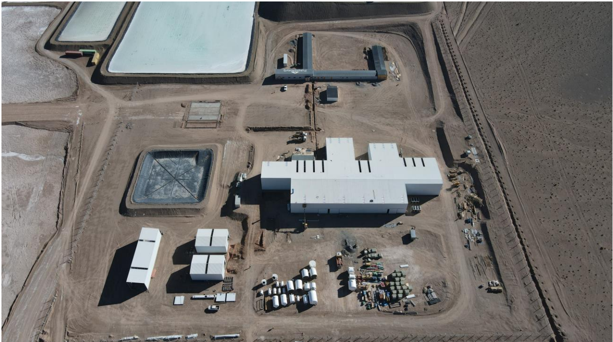
Figure 1. Rincon Lithium Project – 2,000tpa Operation Site Works
