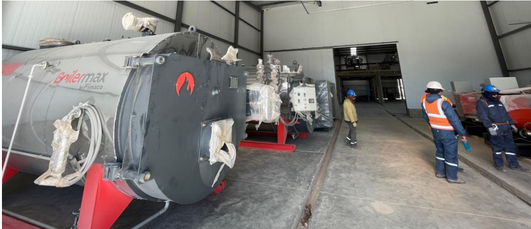
Figure 2. Rincon Lithium Project – 2,000tpa Operation Site Works
