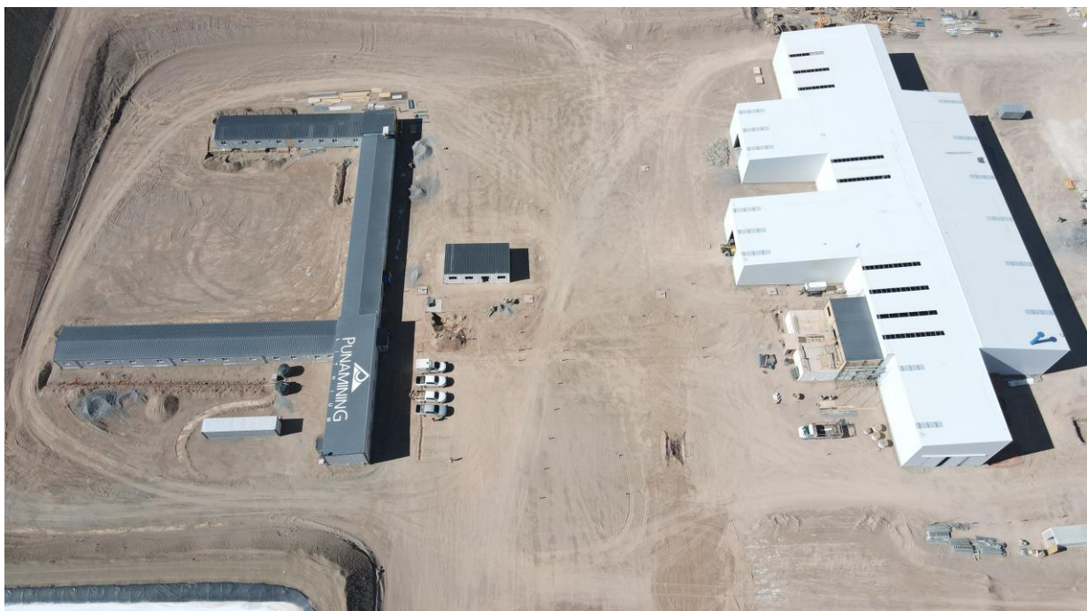
Figure 4. Rincon Lithium Project – 2,000tpa Operation Site Works
