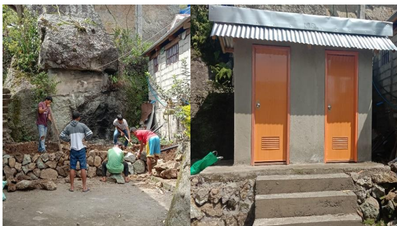
Image 3. Before (left) and after (right) photos of the latrine project.
