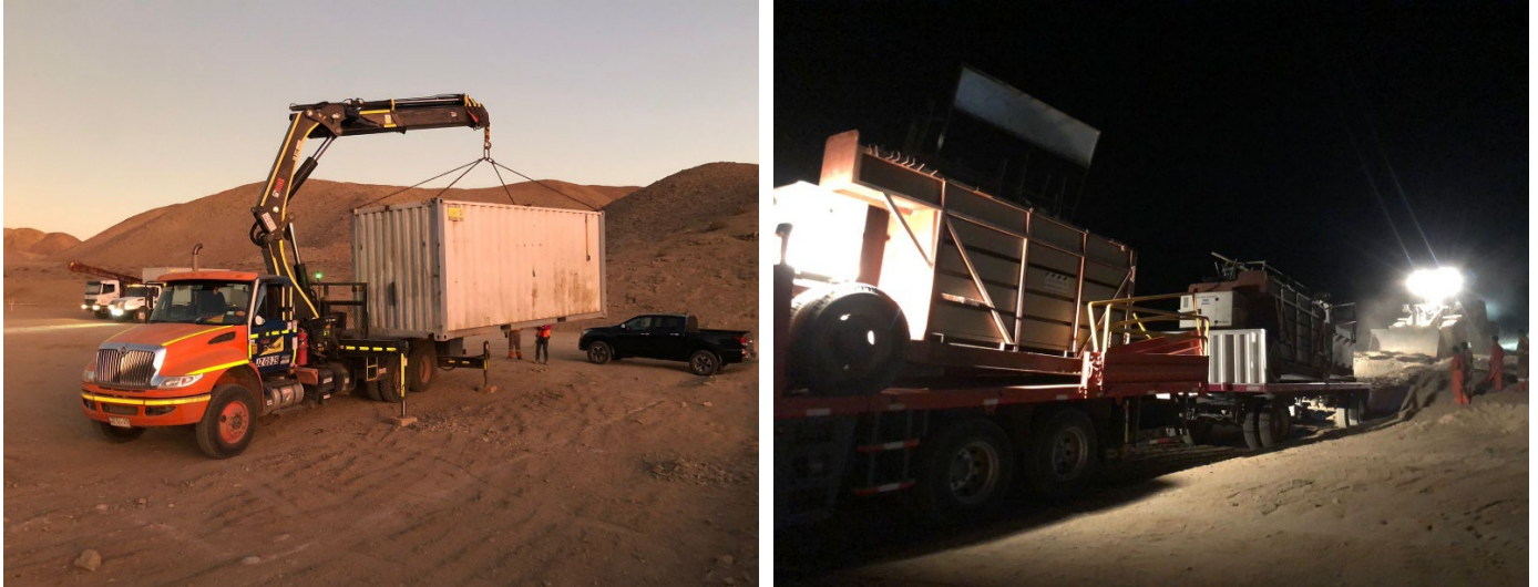
Figure 5 – Drilling equipment arriving on site at El Zorro
