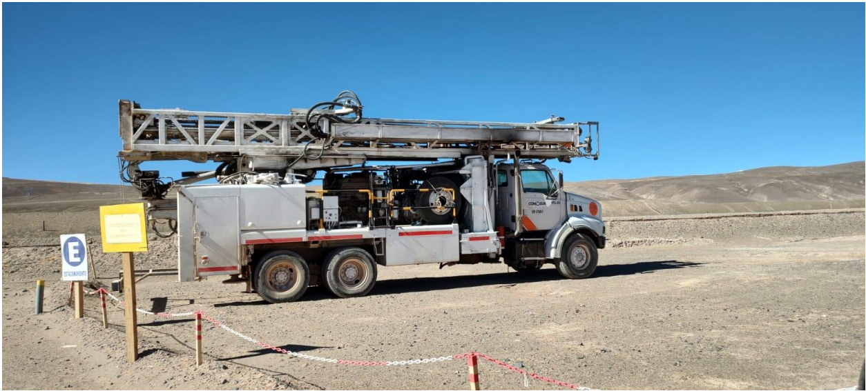
Figure 1. Rincon Lithium Project – Rotary Drill Rig Arriving to Site
