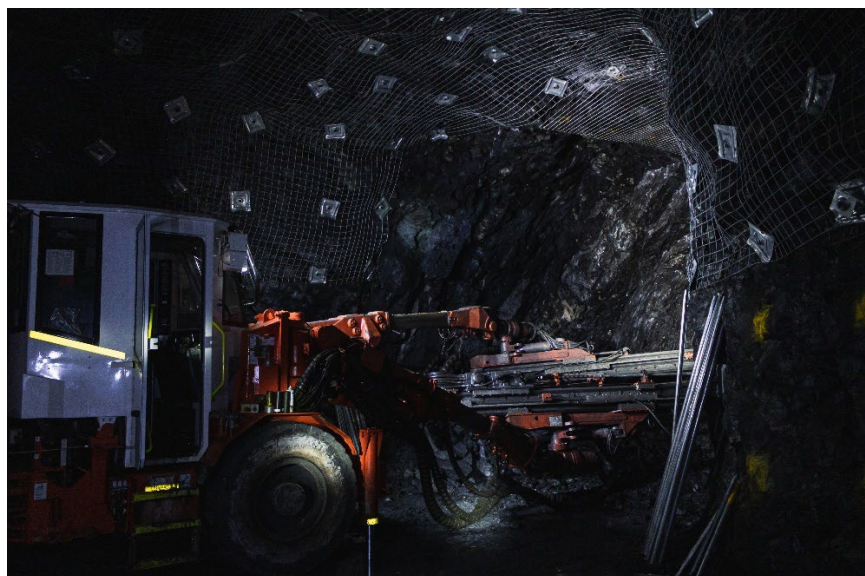
Figure 1. Jumbo undertaking meshing and bolting at Avebury.
