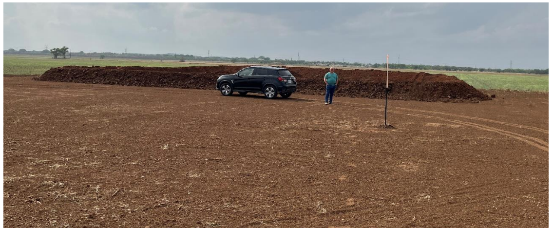
Varn Oil Field - Completed Drill Pad and Pit
