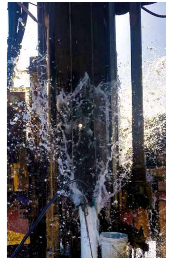
Figure 36: Water pump testing in progress at potential borefield area.
