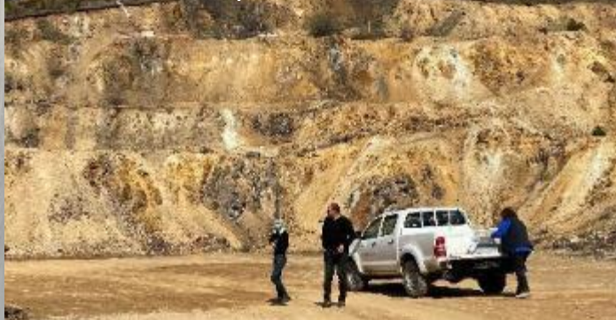
Sastavci O/P mine operated until late 1990s
