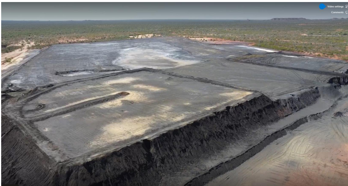
Peko Tailings Dams looking northeast – drone footage
