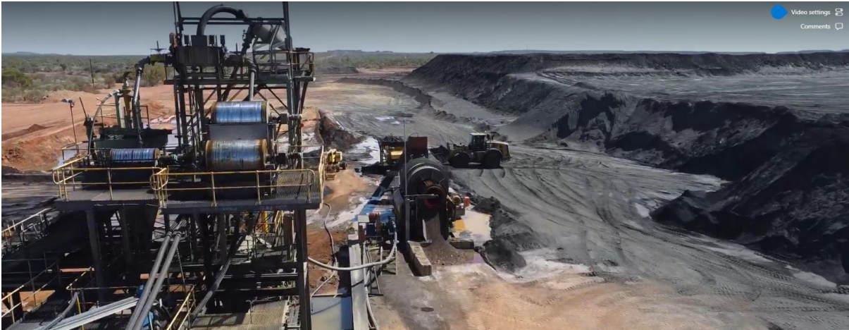
Stockpile material being fed into the plant in background
