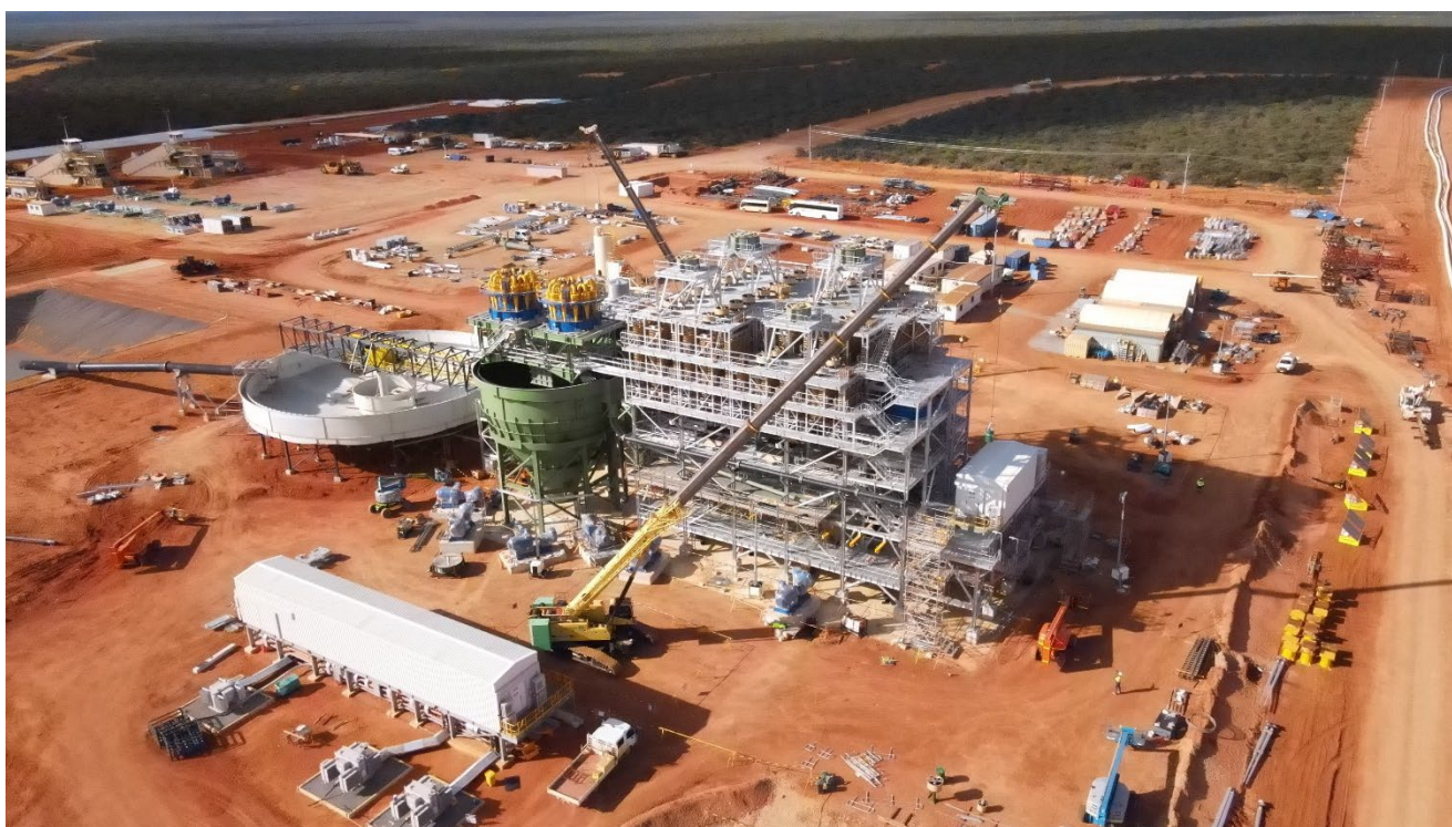
Figure 1 Construction of Coburn’s Wet Concentration Plant progressing rapidly
