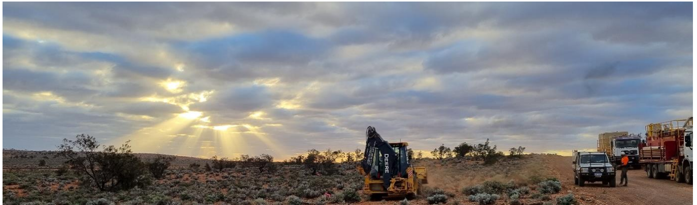
Figure 1 – Site clearing activities at Perseverance West, Tarcoola Gold Project (May 2022)
