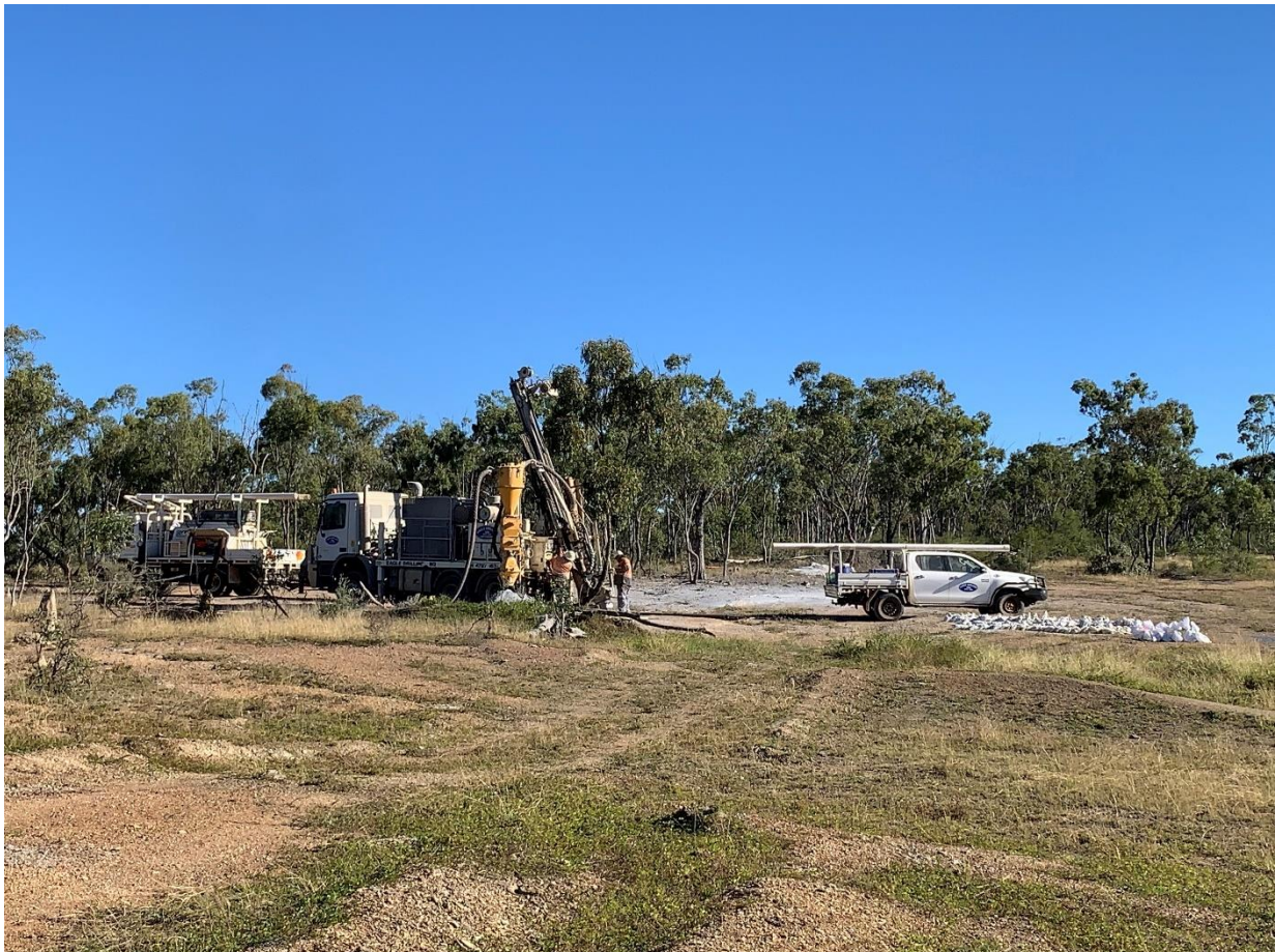
Figure 1 RC drill rig commences drilling at Golden Cup
