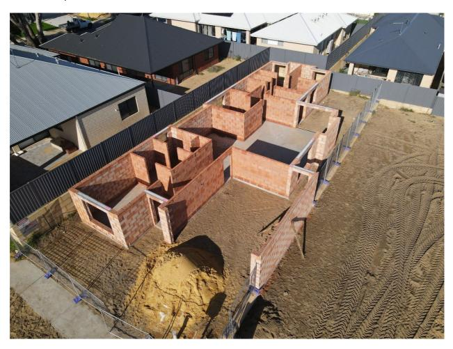
The build utilised two Porotherm block types – R25 double leaf blocks (equivalent in volume to 12 standard bricks) for external walls and single leaf blocks (equivalent in volume to six standard bricks) for the internal walls. This marks the first time in the world Wienerberger's clay blocks have been laid by a robot in the undertaking of commercial, real-world work.
