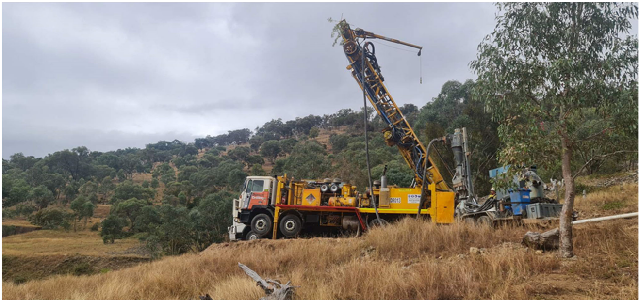
Figure 3: Drilling Rig setting up to drill hole 3DGI003
